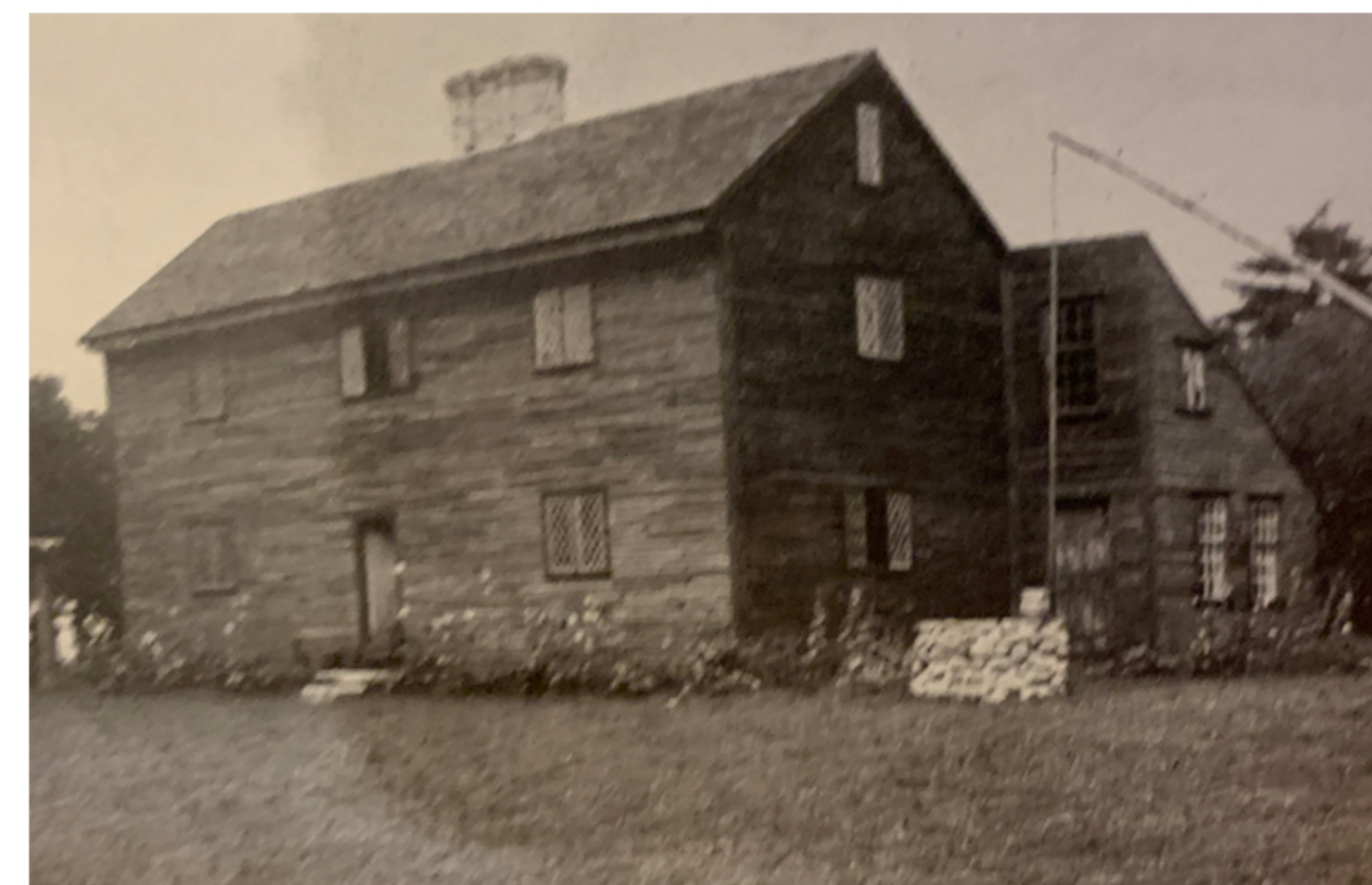
The Goulding house shortly after reconstruction
